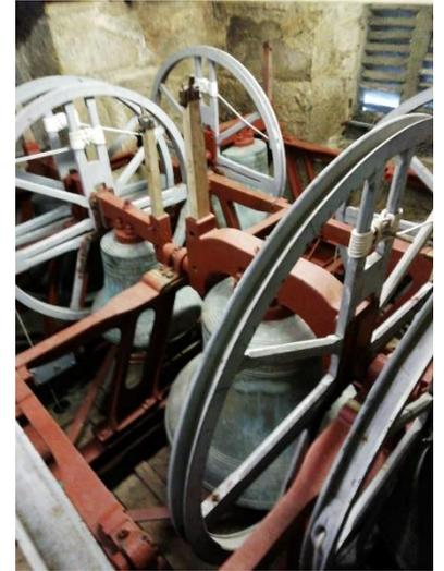
This last bell was the tenor, the largest bell, weighing over 13 cwt or 680kg, and it has the lowest musical note. All these bells were hung on a wooden frame, but that too had to be replaced in 1924. Using cast iron and steel, Taylors were able to fit in two small bells, which they also cast. The smallest, the treble, has the highest note and weighs a mere 3½ cwt or 190kg. Cast into the metal of the treble are the names of the Rector and churchwardens of the time plus the date.
