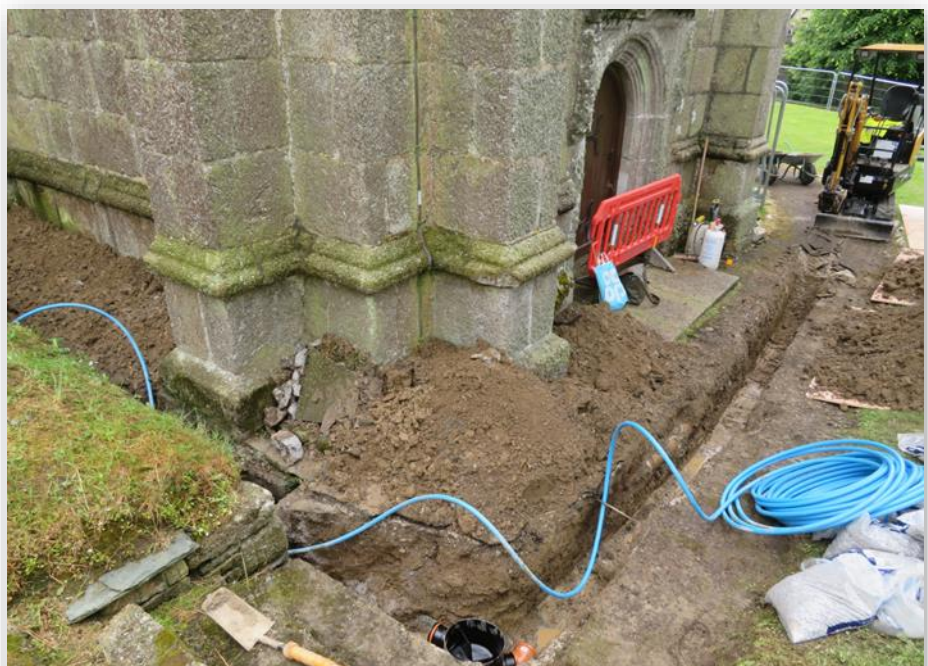
1 Excavation at Lanivet Church north and west wall
